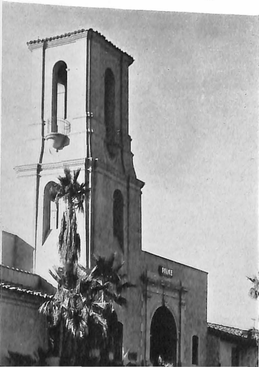
Tower of new Police Administration Building. (Patio shown on pages 36 and 37.)
