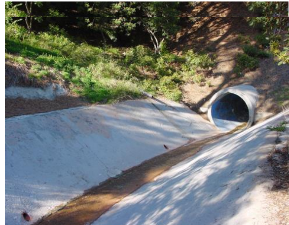
City of San Diego storm drain
