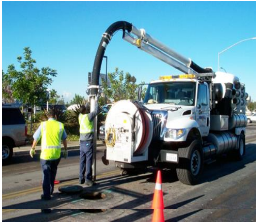
Maintaining the municipal sewer system
