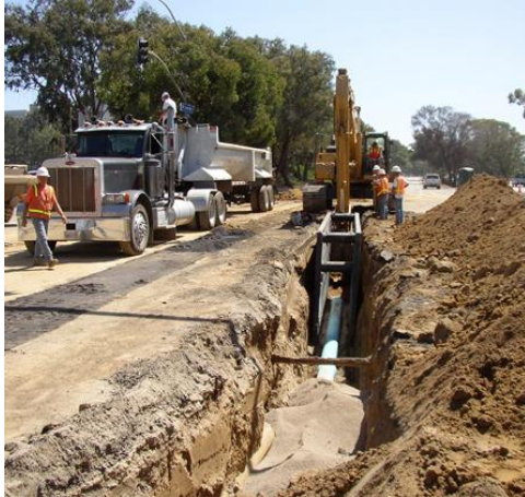
Trenching the municipal sewer system
