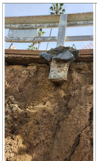
The rail footing exposed, with sidewalk undermining looking up slope.
