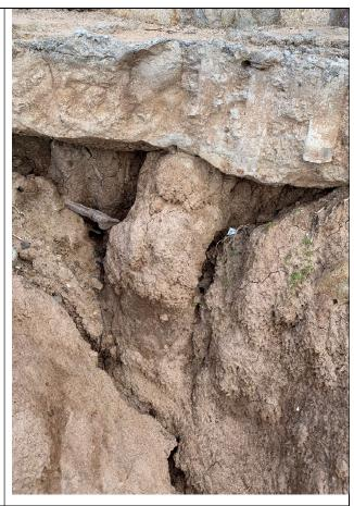
Close up of undermined footing and erosion void below wall
