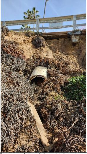
East view of slope failure with 24-inch RCP storm drain exposed.
