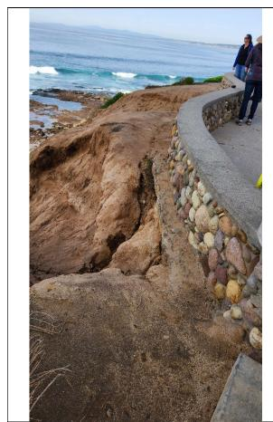
Looking north towards wall footing and slope erosion
