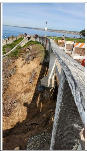
Side view of slope failure within artificial fill placed exposed walkway rail footing.
