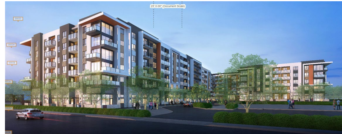
Convoy Square Development Under Construction
