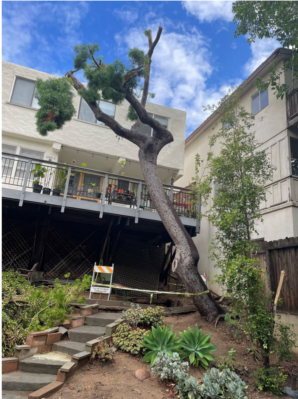
SINKHOLE: PROXIMITY TO TREE AND HOMES
