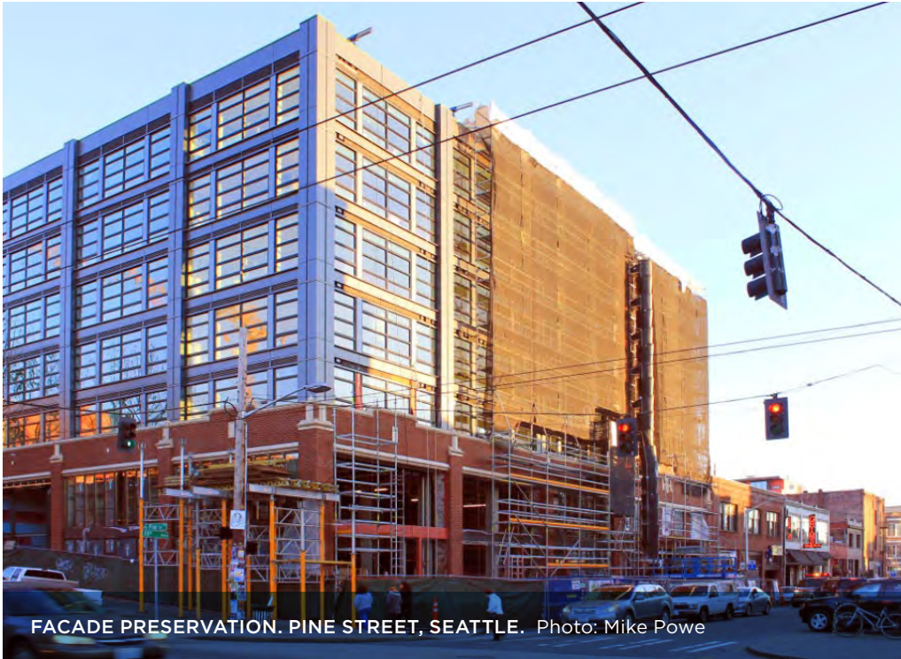
The historic facade from the Sunset Electric building (1916) on Pine Street stands below a nearly-completed 89-unit apartment building.
