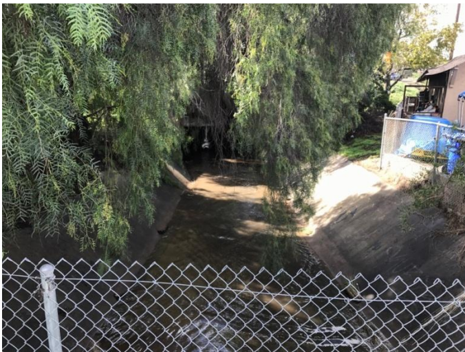
Figure 1: May 2015, looking downstream at concrete channel
