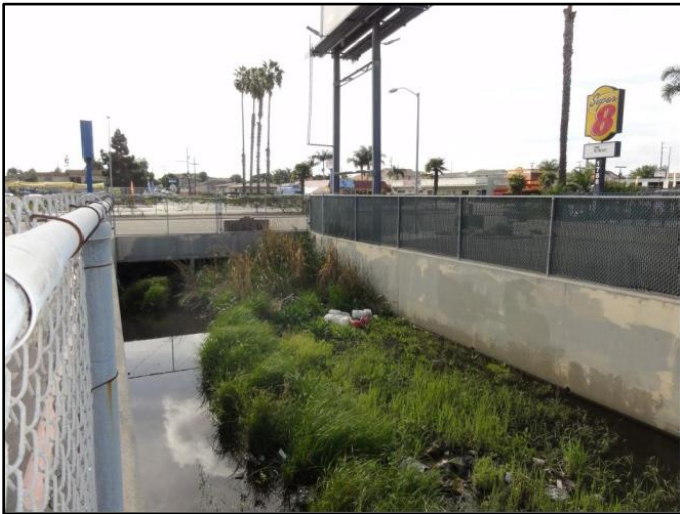
Figure 1: November 2016, looking upstream at the Palm Avenue triple RCB culvert
