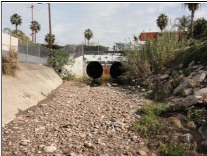
Figure 1: March 2016, looking upstream at the double-barrel 74-inch-diameter RCP culvert
