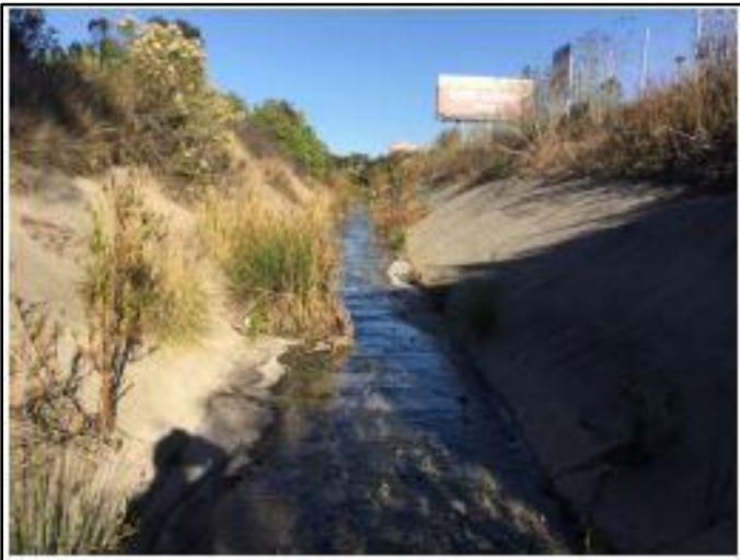
Figure 1: November 2016, looking northeast at the concrete-lined ditch. Note the minimal vegetation established within the ditch.
