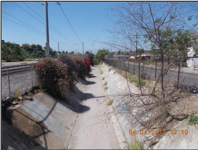
Figure 1: April 2017, looking downstream at concrete channel near 60th Street
