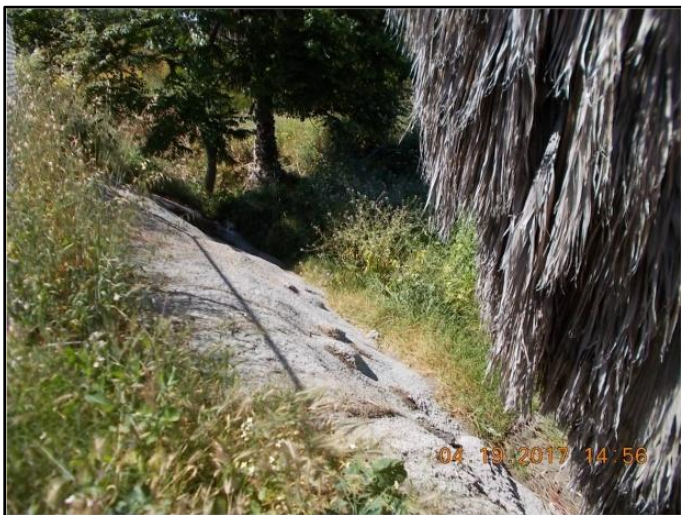
Figure 1: April 2017, looking downstream at vegetation and gunite lining on left bank
