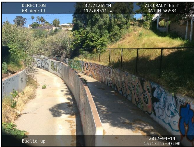
Figure 1: April 2017, representative of concrete portion of channel
