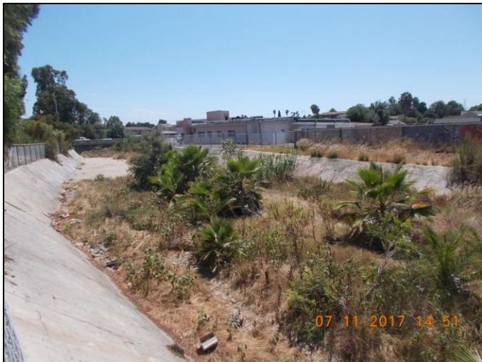
Figure 1: July 2017, looking downstream toward the start of the concrete bottom channel
