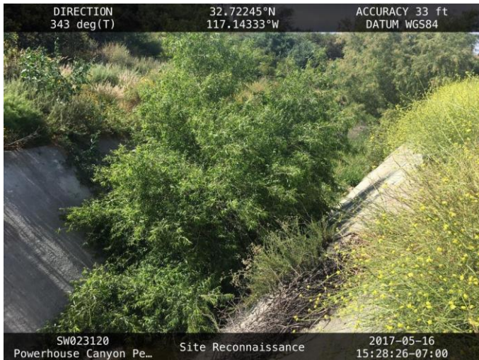
Figure 1: May 2017, looking upstream from the Pershing Drive bridge
