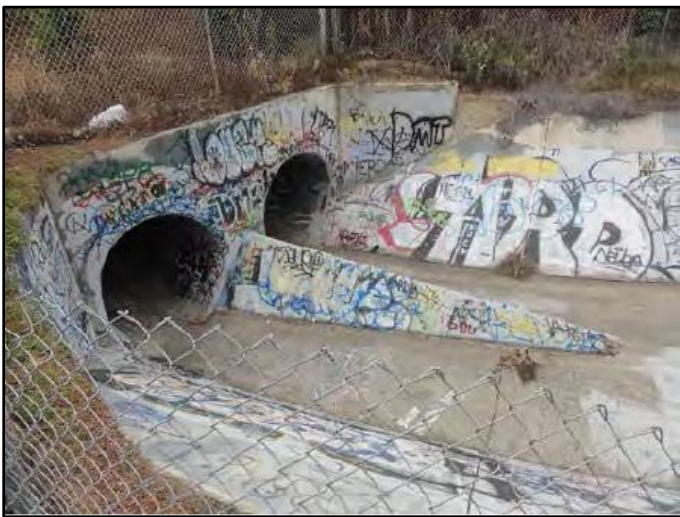
Figure 1: April 2015, entrance to double-barrel 72-inch-diameter RCP culvert under Vista Lane
