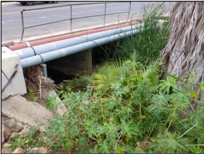
Figure 1: May 2015, looking towards the double 8-foot wide by 5-foot, 2-inch tall RCB culvert at downstream end of segment
