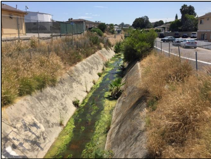
Figure 1: July 2017, looking upstream from downstream end segment
