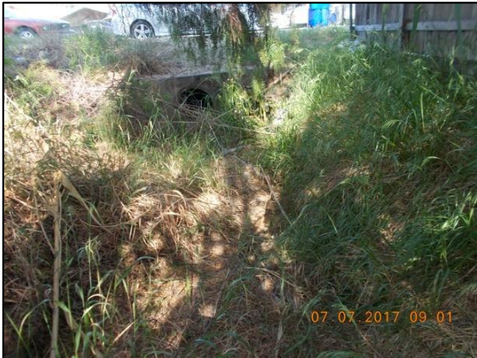
Figure 1: April 2018, looking west at bank repair
