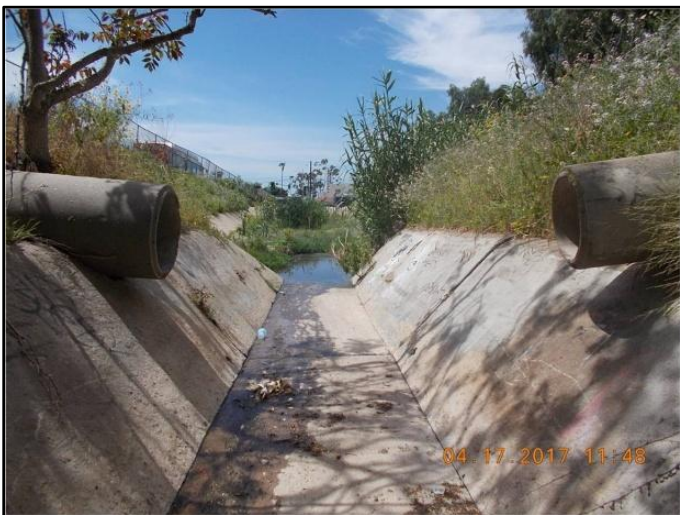
Figure 1: April 2017, looking downstream at transition to Washington 1
