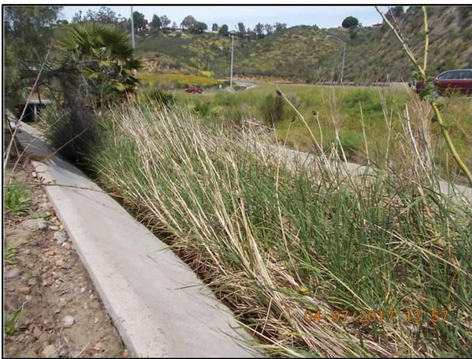
Figure 1: April 2017, looking downstream at vegetation concrete ditch
