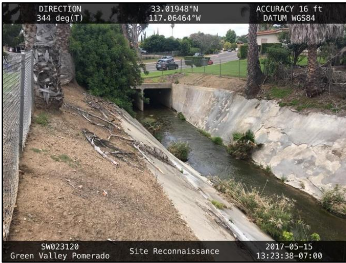
Figure 1: May 2017, looking downstream at double box culvert
