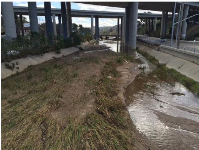
Figure 1: January 2016, looking upstream from the northwest side of the I-5 overpass
