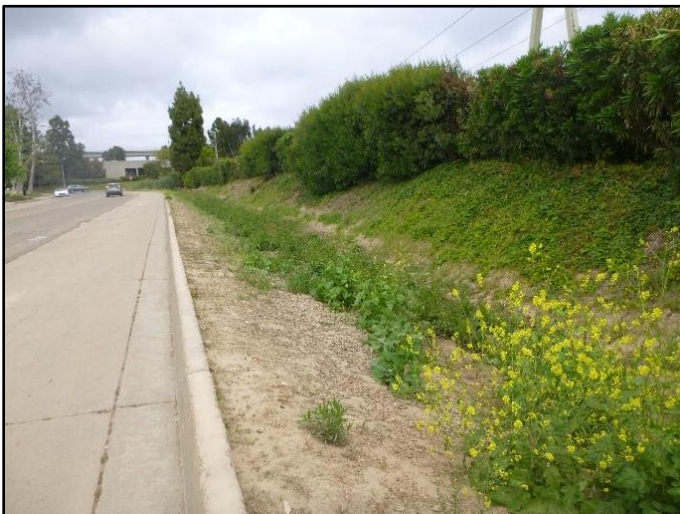
Figure 1: May 2017, looking downstream at vegetation and sediment in Dunhill segment
