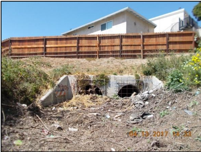
Figure 1: April 2017, looking downstream at dual 54-inch diameter RCP culvert inlet
