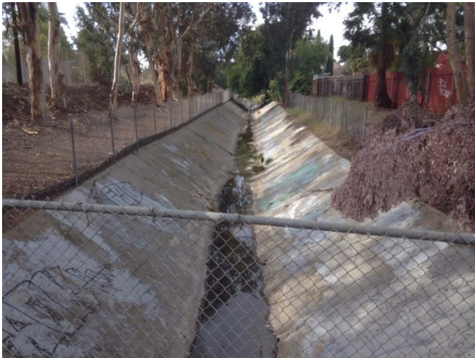
Figure 1: December 2016, above inlet culvert on the Boulder Lake end of channel
