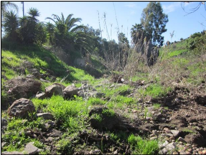
Figure 1: April 2017, looking downstream at sediment, debris, and vegetation
