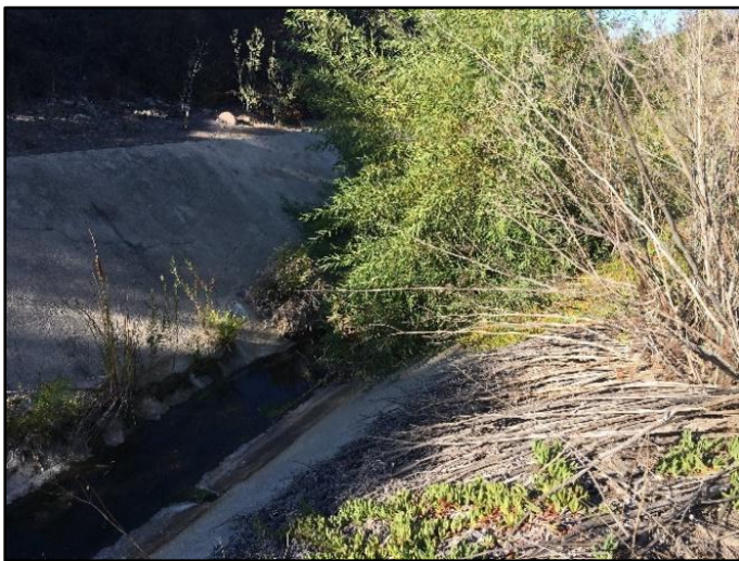
Figure 1: October 2018, upstream of culvert
