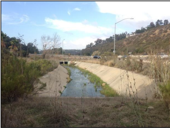
Figure 1: April 2017, looking downstream at concrete channel
