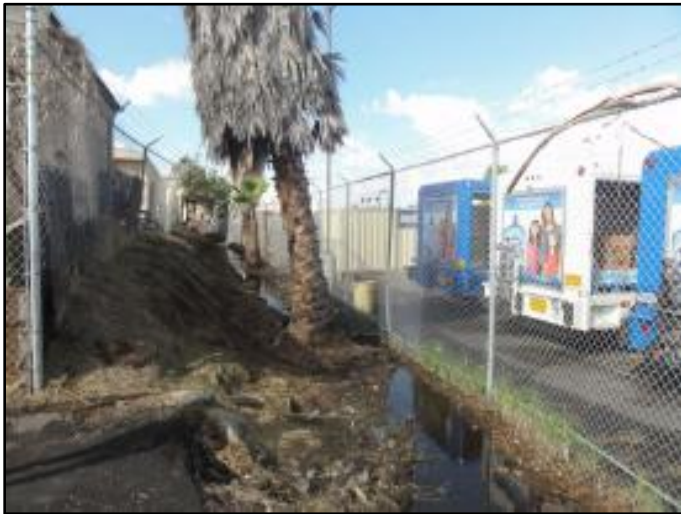
Figure 1: November 2015, upstream portion of reach facing west, showing sediment and vegetation in ditch
