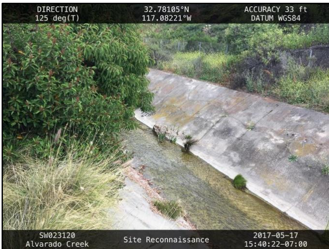
Figure 1: May 2017, looking downstream from the upstream end
