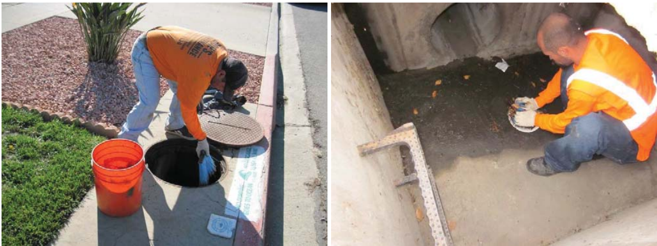
Figure 6. Manual clean-out by Ron's Maintenance in the Tecolote and San Ysidro areas.
