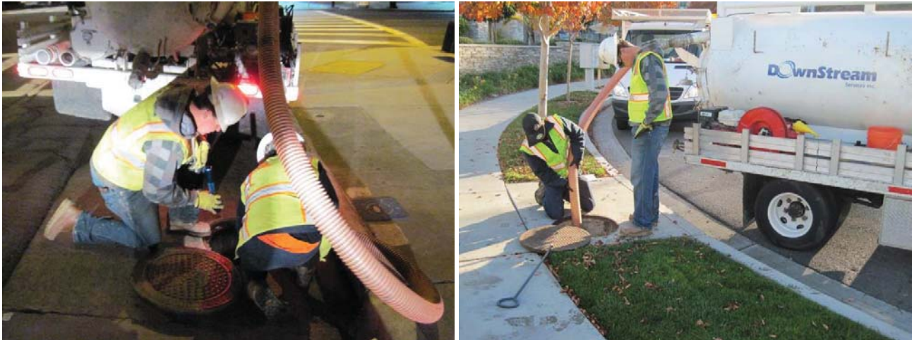
Figure 7. Vactor clean-out by Downstream Services, Inc. in the Downtown and Poway areas.
