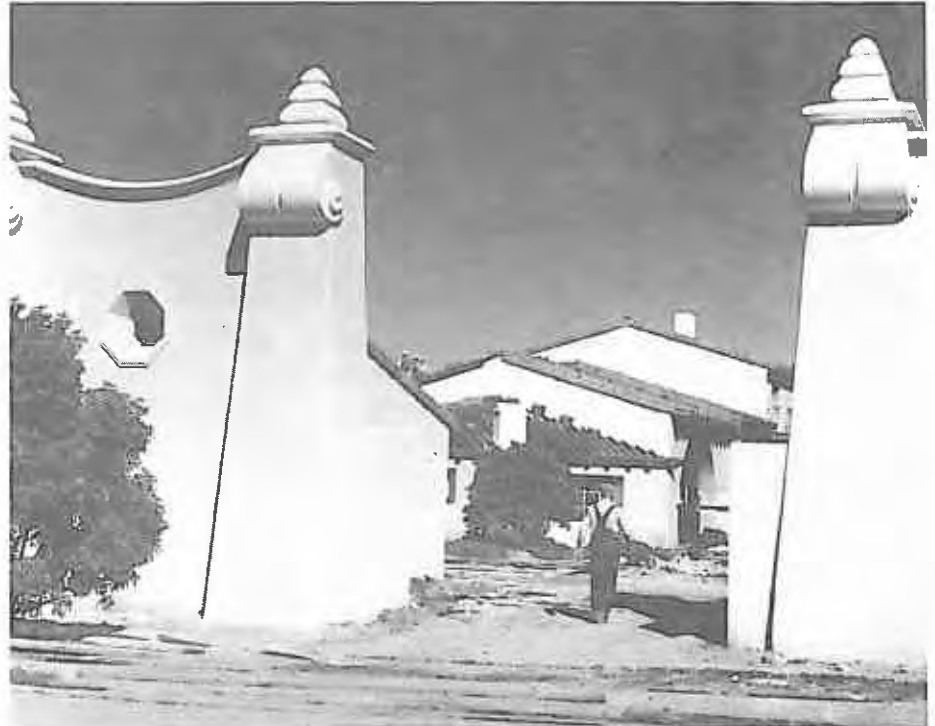
The south entry of Spanish Village with a view of the Central building during construction in 1935.
