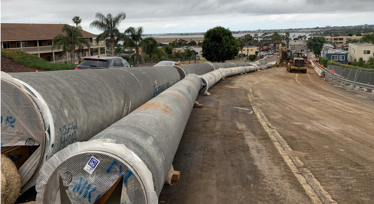
Morena conveyance pipelines
