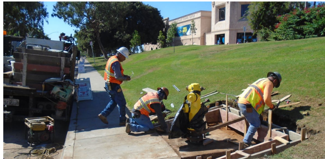
Water pipe installation at Balboa Park
