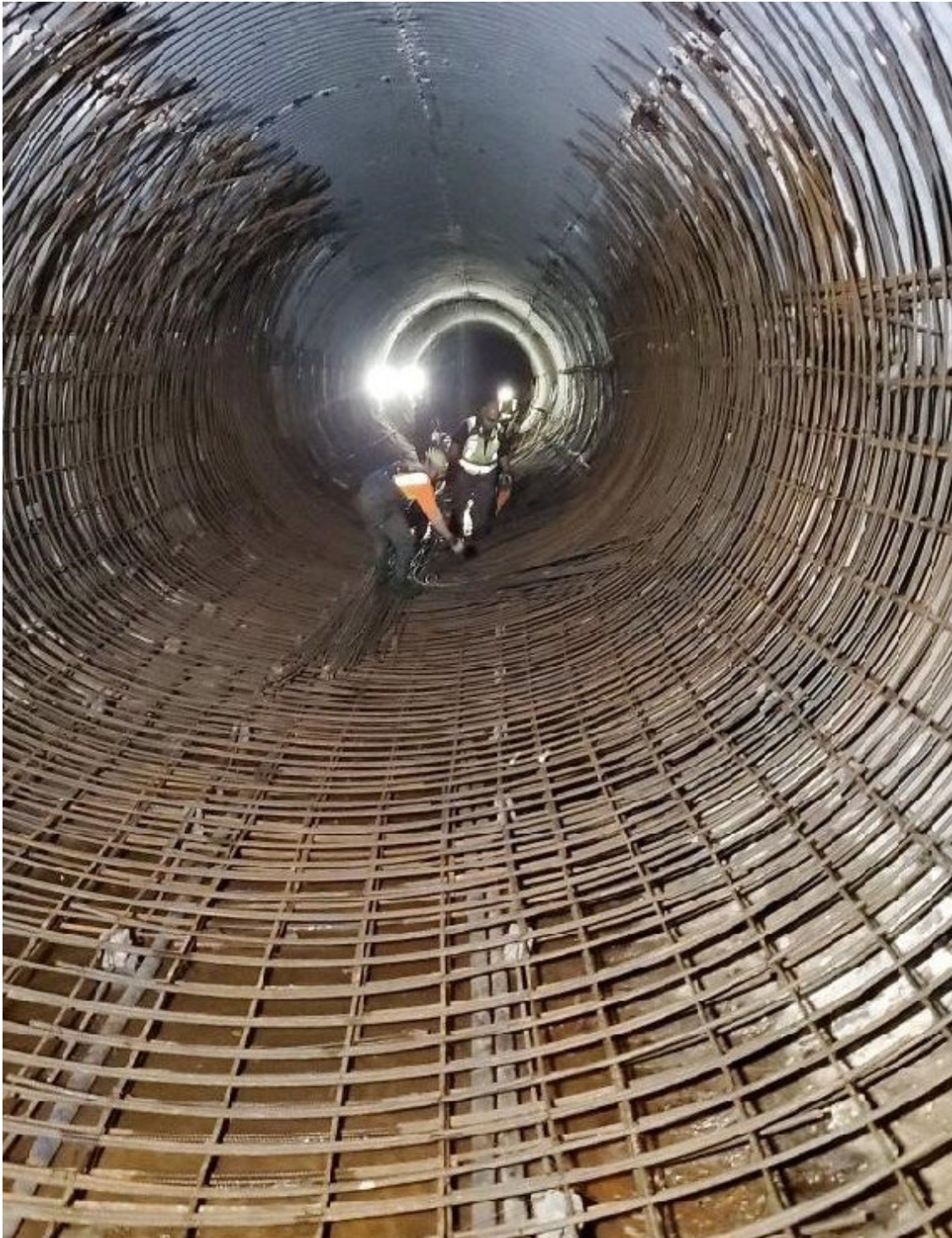
Villa La Jolla Storm Drain Emergency Repair Project construction
