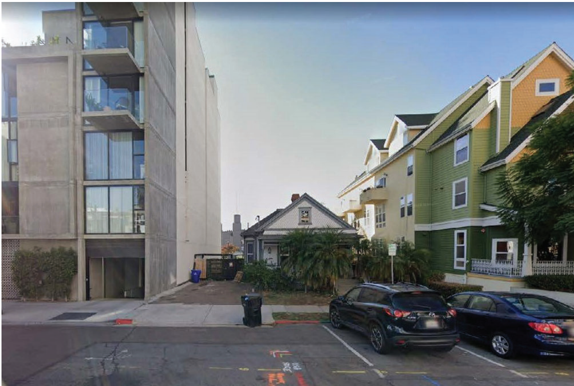
Figure 5-3: Looking west at the Andrew Cassidy Home located between two multifamily residences. Source: Matthew Segal.
