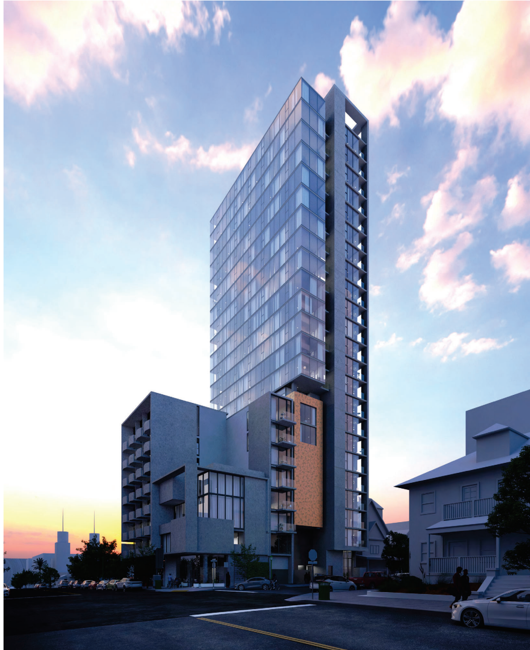
VIEW FROM WEST CEDAR STREET LOOKING WEST
