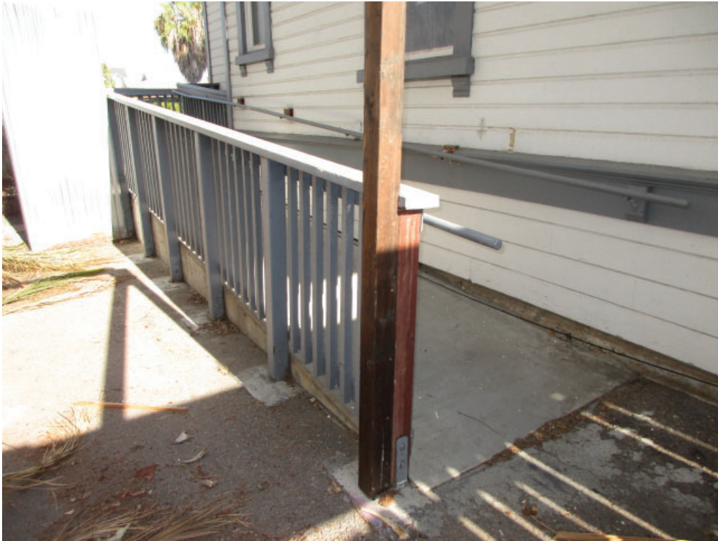
Figure 3-13: Looking northwest at the accessibility ramp located at the south facade. The ramp is a combination of cast-in-place concrete and OSB wood boards.
