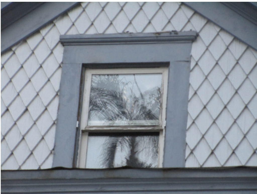
Figure 3-6: Looking west at the gable end of the east facade showing the diamond shaped wood shingles and replacement double hung window.
