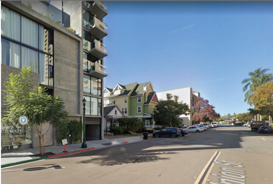
Figure 5-1: Street view looking northwest along Union Street. The Andrew Cassidy Home is located at the west portion of the street barely visible between two multifamily residential properties. Source: Google Maps.
