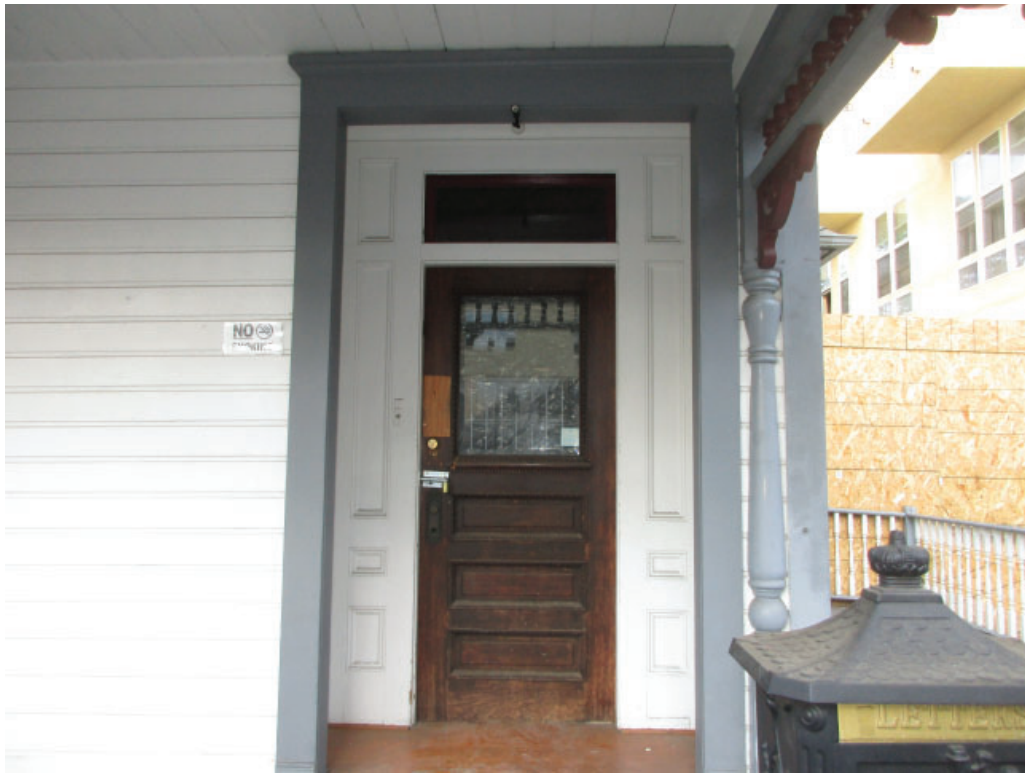
Figure 3-9: Detail view showing the original three panel entry door with glazed lite and fixed wood transom window above. The original door hardware is missing.
